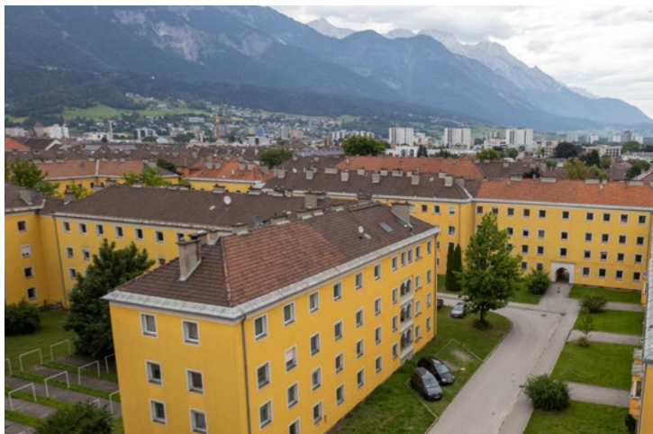
The Eichhof district, photo: M. Freinhofer
